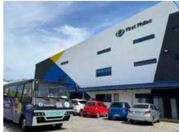
First Philec, Inc.'s (FPI) as a solution's provider for power distribution
